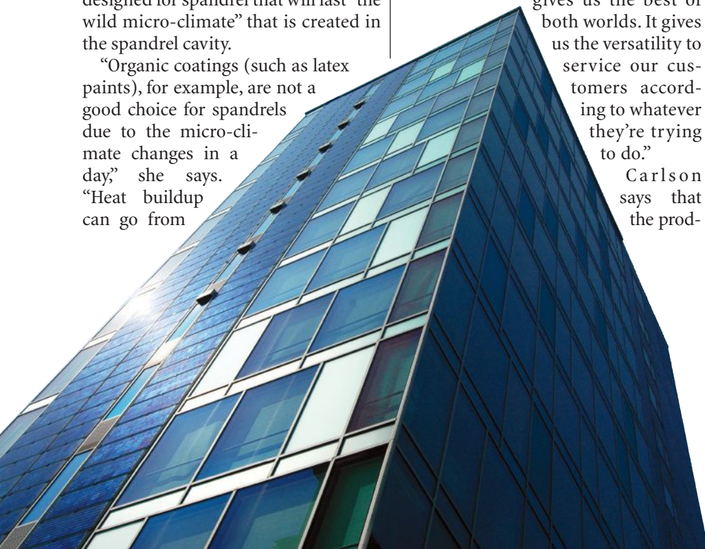
Ceramic frit and silicone coatings are still the prominent products used to make spandrel glass opaque.
