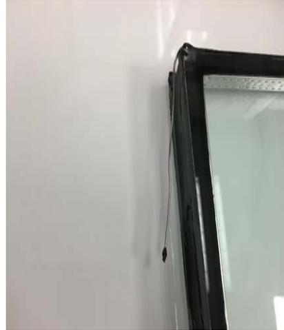
Figure 2: Apply silicone dab to tube end
