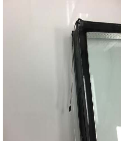
Figure 2: Apply silicone dab to tube end
